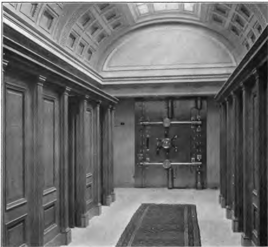
Safe Deposit Room and Vault.
